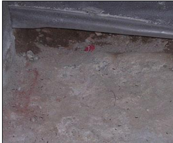
Detall possible mur perimetral UE 829
